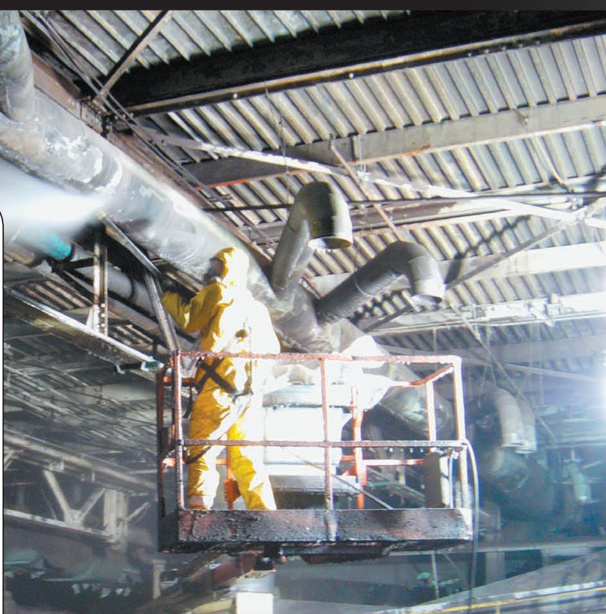
A crew member power washes contaminated material inside the the foundry
