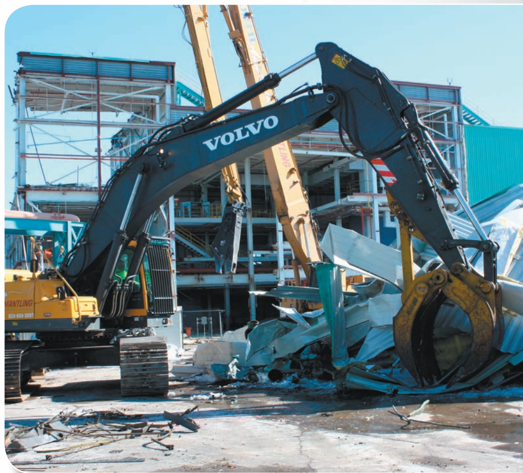
A Volvo EC460 hydraulic excavator uses a grapple to process material for recycling.
