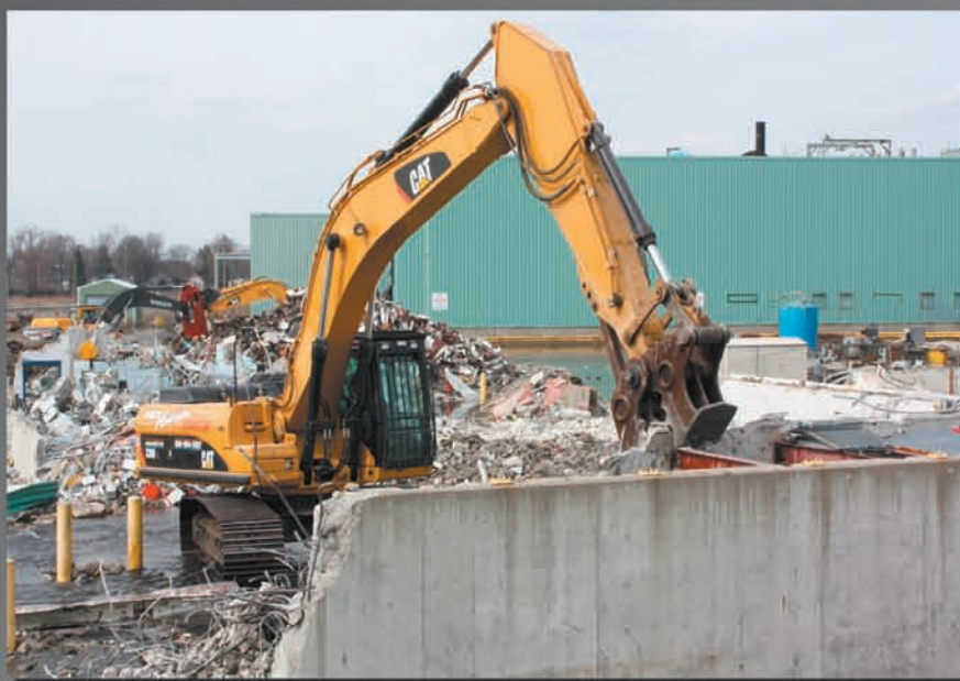
Controlled demolition of concrete structures using a CAT 330DL excavator with a concrete pulverizer.
